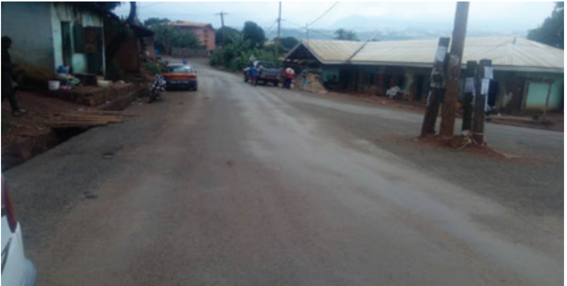
Newly constructed road, Bamenda II Zone, 2018
